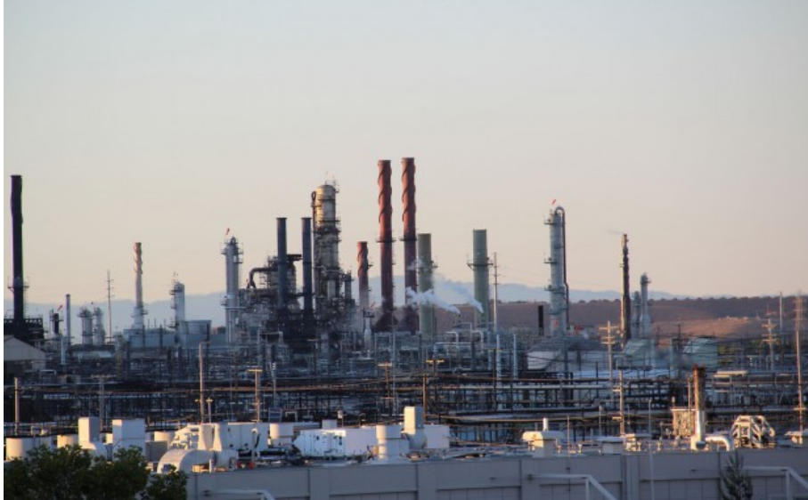
Part of Chevron's expansive Richmond refinery. (Photo by Rachel Waldholz)
